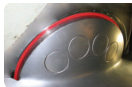
Step 6: Installed seals for runner blades
