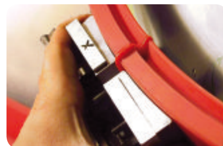
Step 3: Welding of aligned cross sections
