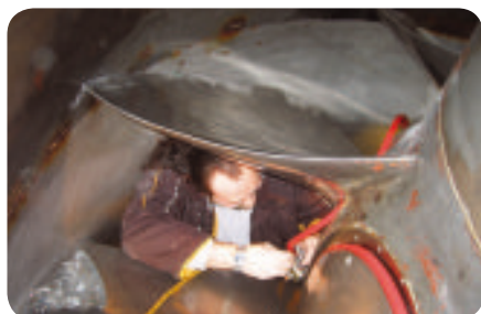
Step 1: Mounting of runner blade seals
